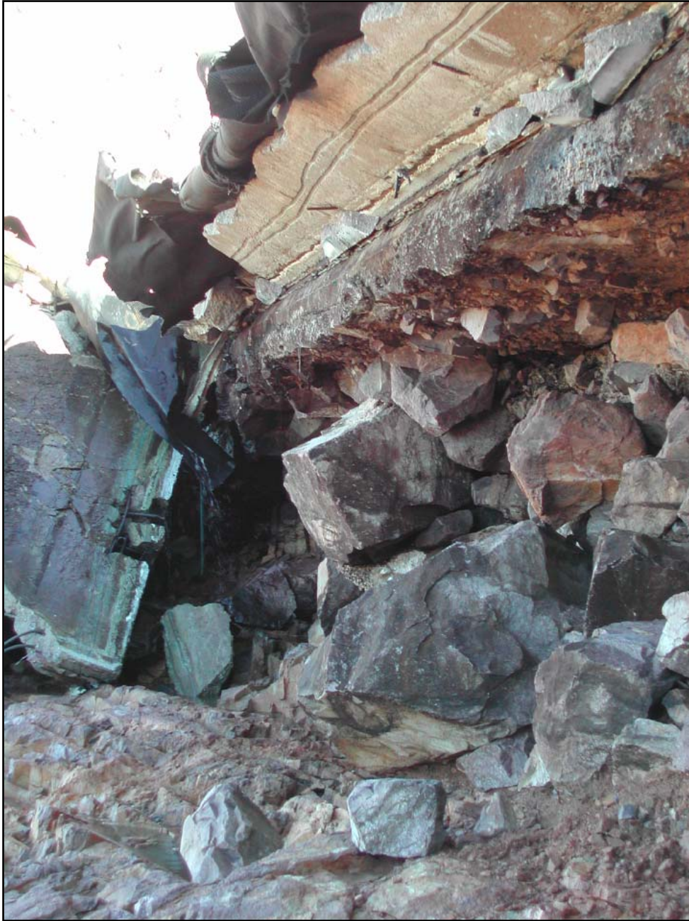
Rockfill between top of rock and base of plinth
